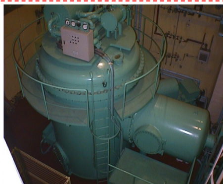
Electron accelerator (0.5~2.0 MeV 0.1~30 mA)
