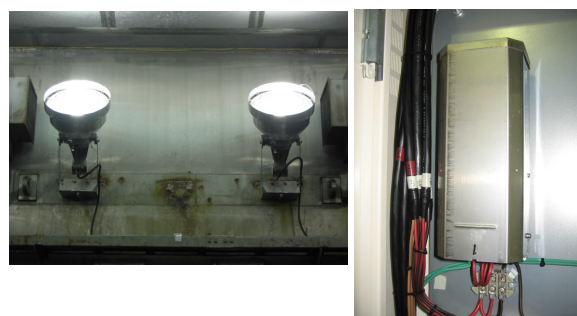
Fig. 2 Radiation-resistant lightings (left side) and ballast (right side).
