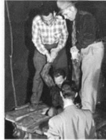
Figure 5 Dr. Frederick Reines (left) and Dr. Clyde L. Cowan (right), co-discoverers of the neutrino, lower a fellow worker into the first "whole body counter", the scintillation assembly used in their experiment. Reines, Dr. Wright Lambam, inside the counter, peers from the opening.
