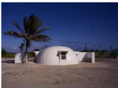
Figure 3. The newly constructed radiological facility on Eniwetok Island—this "igloo" design is a low maintenance facility ideally suited to withstanding high wind and harsh sea salt environments.
