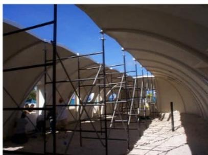
Figure 2. Construction of the modular shell sections utilizing internal scaffolding.
