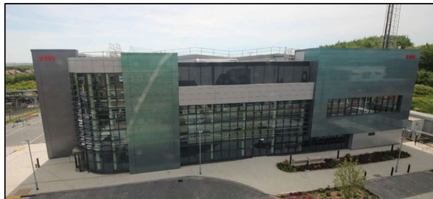
Fig. 1 Extreme Photonics Applications Centre building at the CLF, UK.
