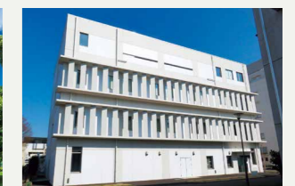
Advanced Radiation Medical Dosimetry Building
