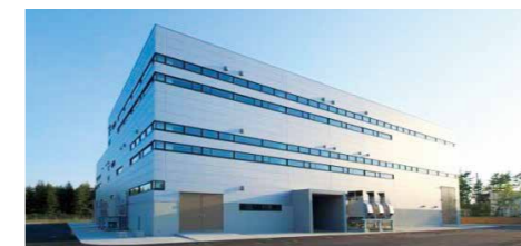
Blanket Test Facility Building
