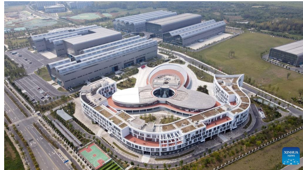
Comprehensive Research Facility for Fusion Technology (CRAFT) in Hefei, east China's Anhui Province
