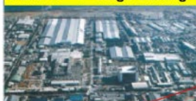
FEIC: 1st-4th stage cabling
