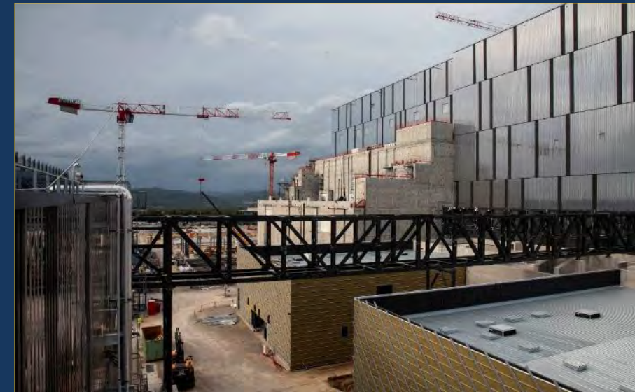
▶ Bridge to support cryolines between Cryoplat and Tokamak Bldg.
