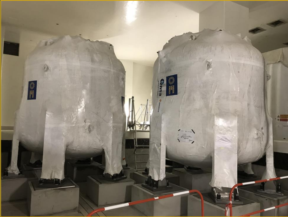
October 2021: Installation of 12m 3 Water Detritiation water storage tanks
