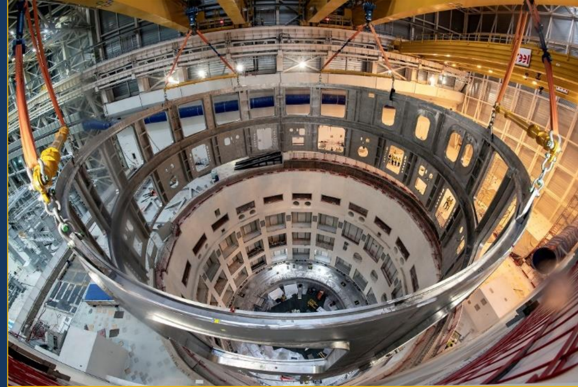
Inserting the Cryostat Lower Cylinder into the Tokamak Pit. Perfect fit with the Base 31 August 2020
