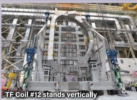
Installation of first sector sub-assembly
