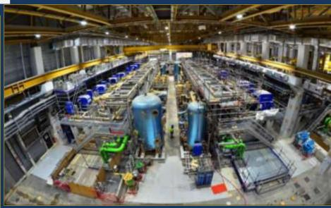
Close to 5,000 tonnes of equipement are now installed in what will be the largest cryogenic unit in the world, tasked to provide the cooling fluids to the magnetic system, cryopumps and thermal shield. Work is now ~ 50% complete.
