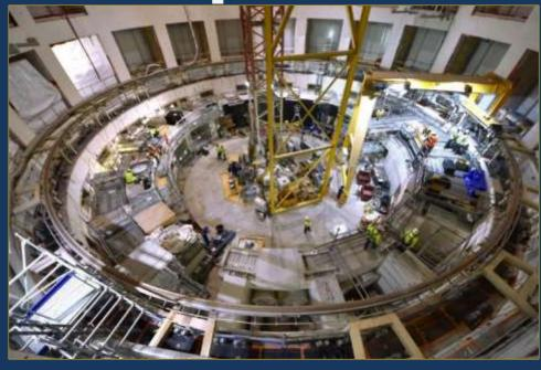
Civil works for the main building (Tokamak Bldg) are completed. Work is ongoing for the extension of the crane rails and the creation of the Crane Hall. Inside the Assembly Pit, anchoring systems are being installed on and around the "crown" that will support the combined mass of the machine and its enveloping cryostat (23,000 tonnes).
