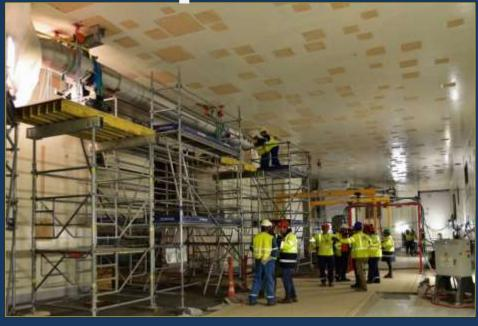
Manufactured partly in India and partly in France, some 2.7 km of high-technology piping ("cryolines") must be assembled and welded inside the Tokamak building to distribute cooling fluids to the magnets, thermal shield and cryopumps. Installation works began in September 2019.
