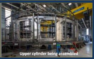
Manufactured in India, the 30 m x 30 m cryostat (the insulating vacuum vessel that encloses the machine) is being assembled and welded on site by German company MAN Energy Solutions. The lower cylinder is in storage; the base section is finalized; assembly work has begun on the upper cylinder.
