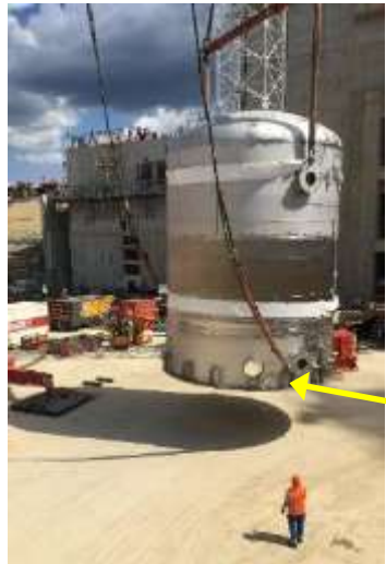
Installation of Drain Tank
