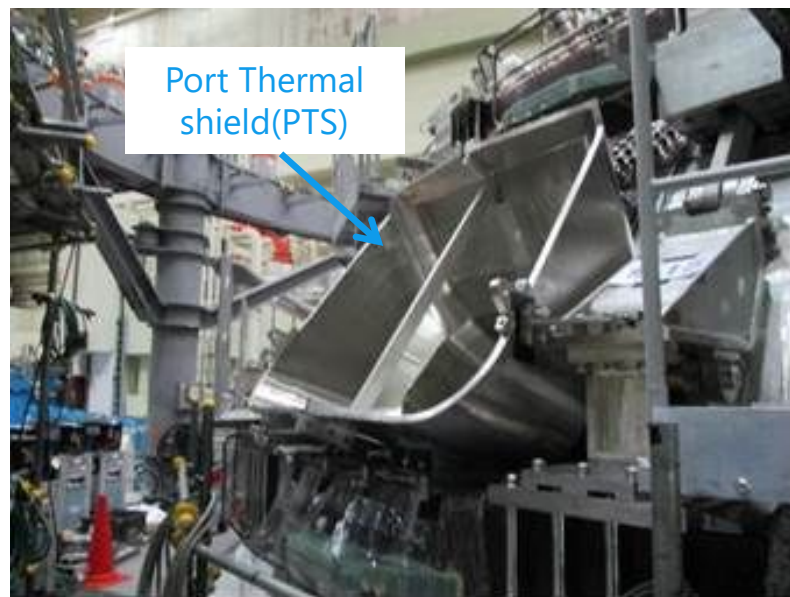
Assembly of Port thermal shield
