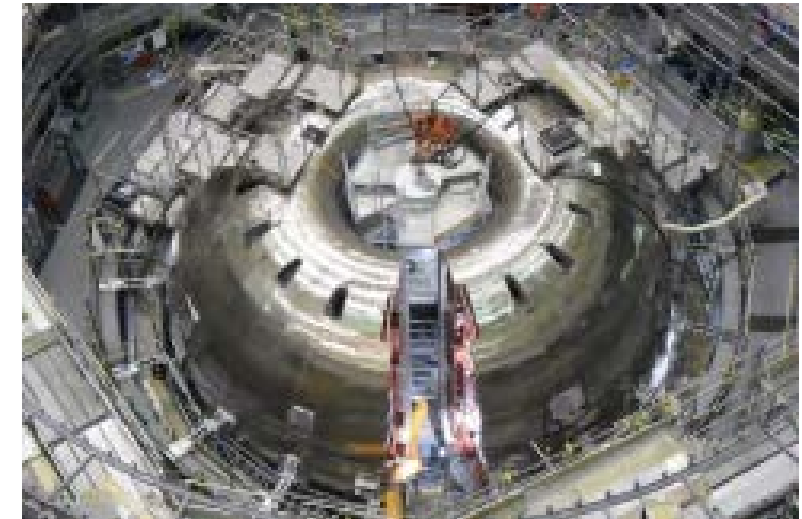
Completion of welding of 340° VV
