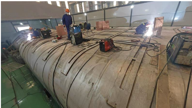
April 2025: bottom support welding ASIPP/SENPEC (China)
