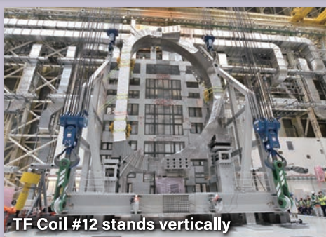
Installation of first sector sub-assembly
