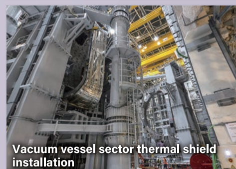
First sub-assembly completed
