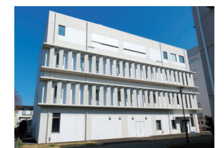
Advanced Radiation Medical Dosimetry Building
