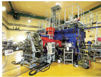
Ion Irradiation Research Facility TIARA (in service)
