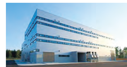
Blanket Test Facility Building
