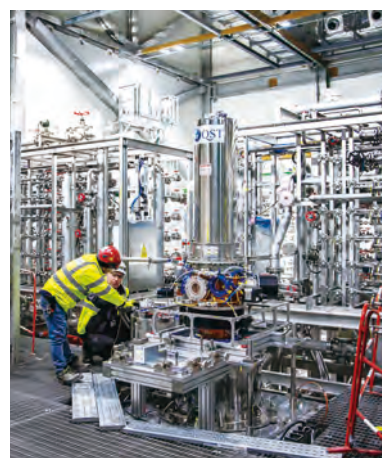
Installation of the gyrotron RF heating device procured by QST/JADA
