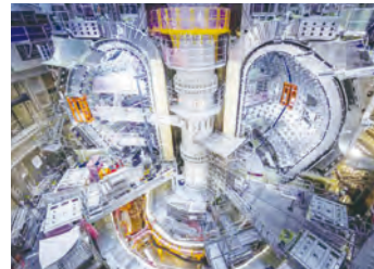
Inside the tokamak pit where a total of five sector modules are installed
