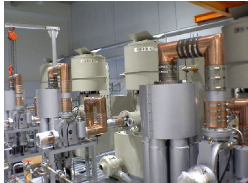
200 MHz transmitters (200 kW x 4, from JFT-2M)
