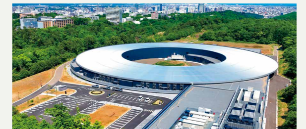
3 GeV Synchrotron Radiation Facility NanoTerasu (for sharing according to the Act on the Promotion of Public Utilization of the Specific Advanced Large Research Facilities)
